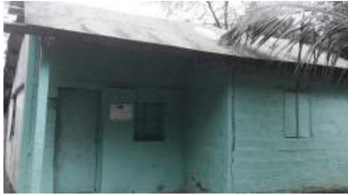
Cast in-situ Ferrocement Roof
