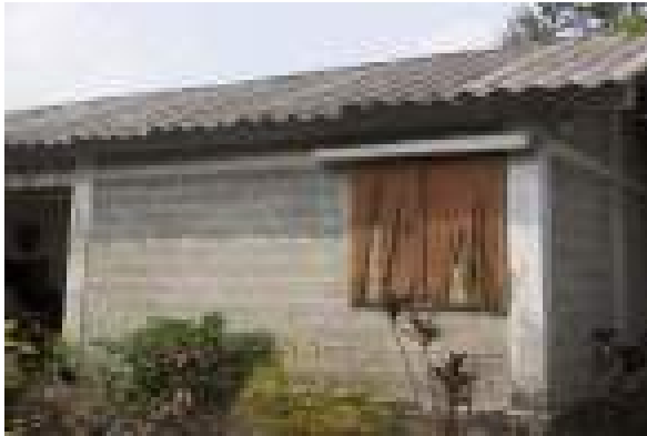
Ferrocement Corrugated Sheet
