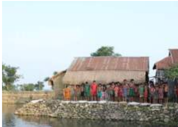
Protection with retaining walls and stones
