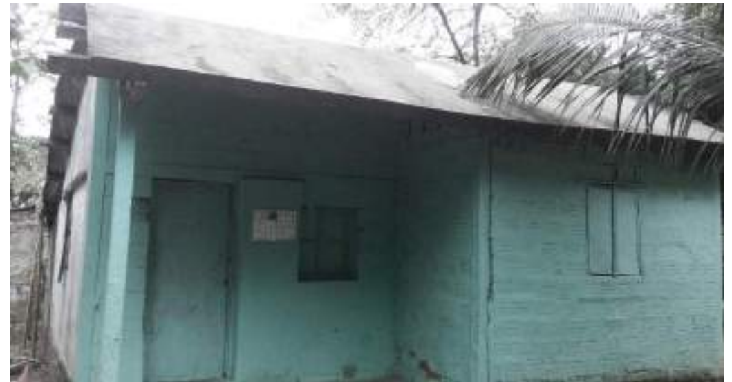
Cast in-situ Ferrocement Roof
