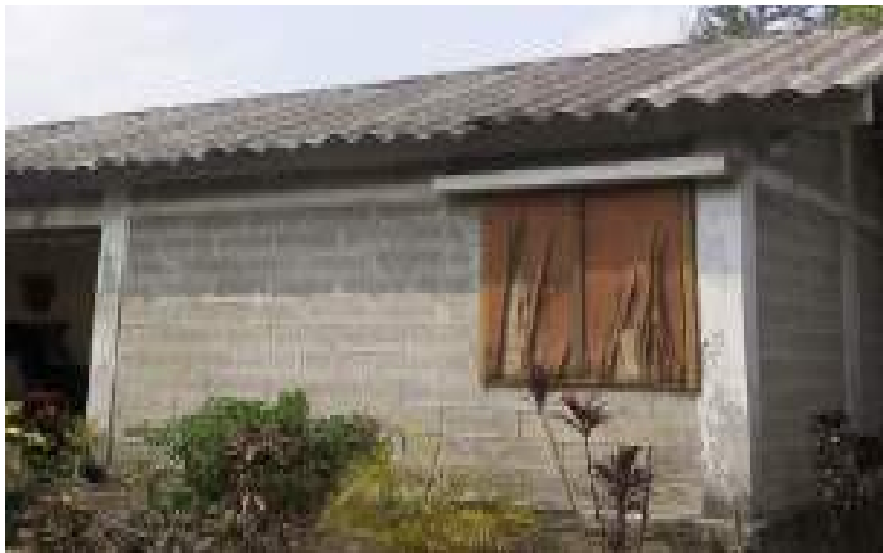
Ferrocement Corrugated Sheet
