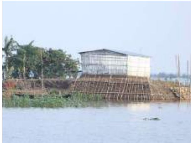
Protection with local stone and bamboo
