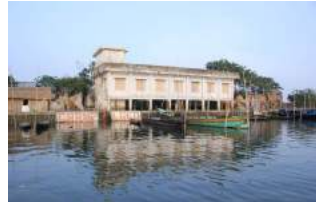
Protection with retaining wall
