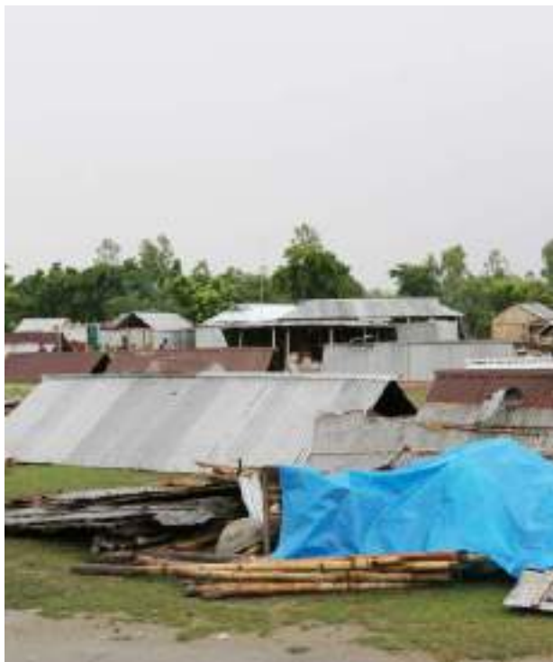
Household damaged by storm
