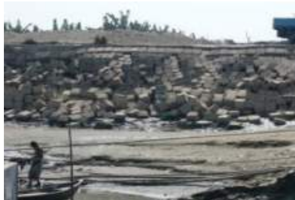
Concrete slope-stabilization blocks
