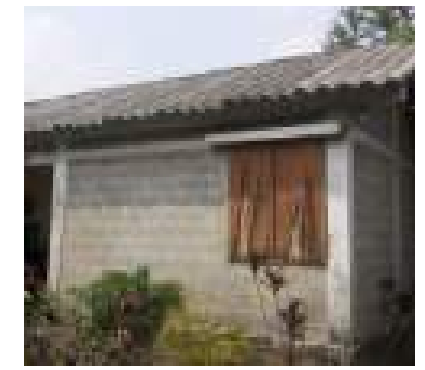
Ferrocement Corrugated Sheet
