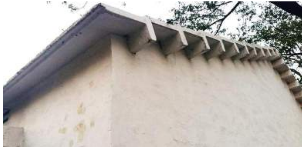
Ferrocement L-Panel
