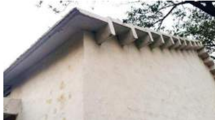
Ferrocement L-Panel
