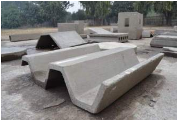
Ferrocement Folded Plate
