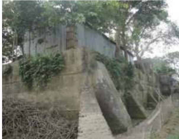
Protection with retaining walls along with buttresses
