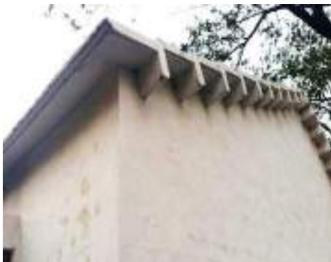
Ferrocement L-Panel
