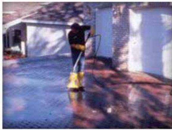
Figure 2: Pressurized cleaning equipment used by professional cleaning and sealing companies can bring out the best appearance from pavers
