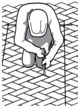
Figure 2. Removing joint sand surrounding the first paver to be removed.
