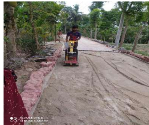
Figure: Compaction of Base
