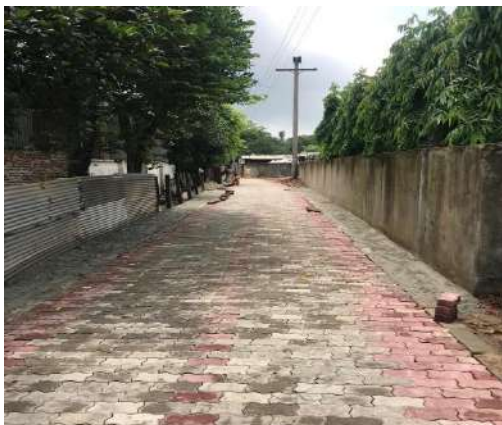
Figure: Completed Roadway
