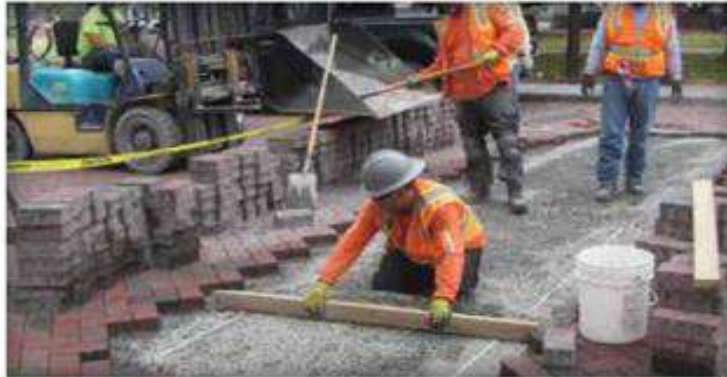
Figure 2. After compaction of the base, bedding material is screeded.
