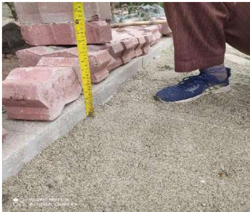
Figure: Measuring and Checking the level of Base
