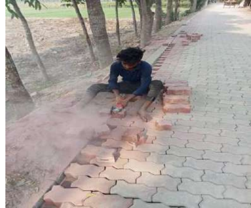
Figure: Cutting and Laying in Stretcher Bond for adjustment with curb stone
