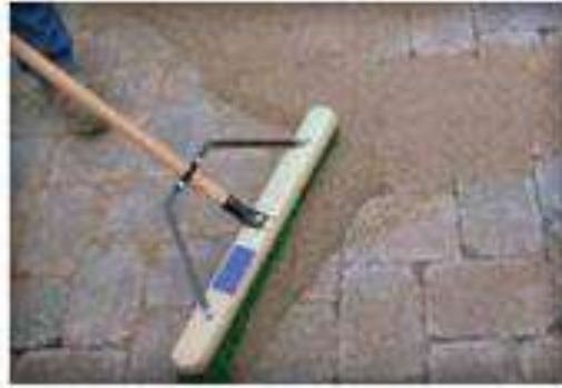
Figure 5. Joint sand can be pre-mixed and delivered to the site (typically in bags), or mixed with stabilizer at the site, then swept into the joints, compacted for consolidation in them to create interlock, and wetted to activate the stabilizer.
