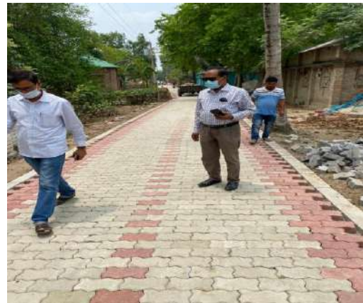
Figure: Ongoing Designed Block Laying
