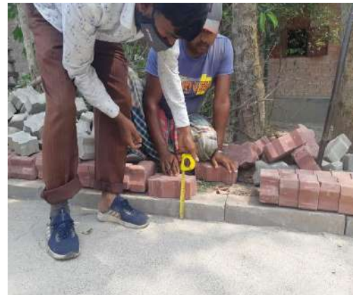
Figure: Measuring and Checking the level of Base
