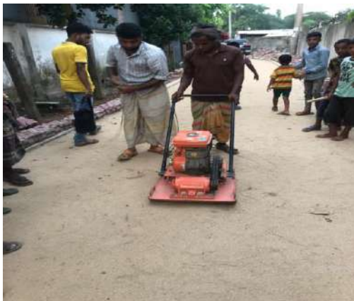
Figure: Compaction of Base
