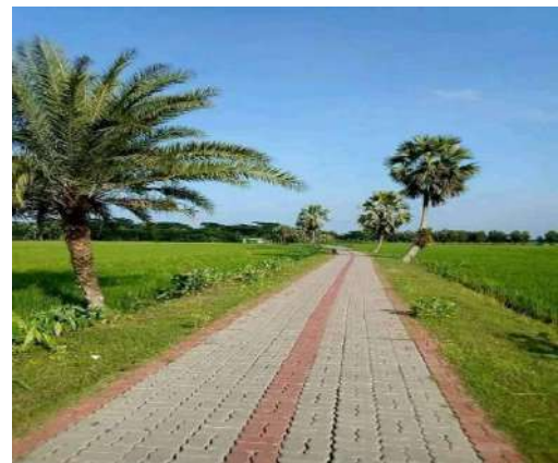
Figure: Completed Roadway
