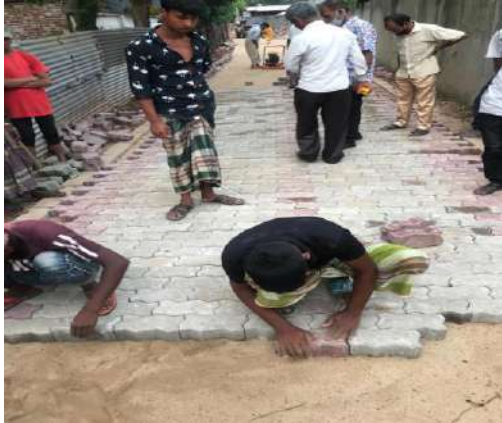
Figure: Block Laying in Stretcher Bond
