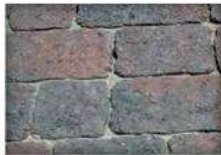
Figure 4. Liquid joint sand stabilizers can deepen the surface color slightly and they provide some surface sealing as well. Tumbled pavers shown here have wider joints than other shapes. These type of pavers can require stabilization of the joint sand.
