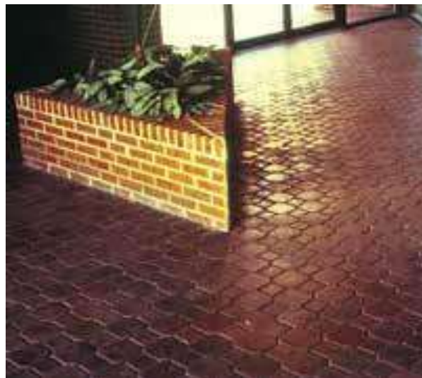
Figure 1: Many sealers enhance the appearance of concrete pavers and protect against staining
