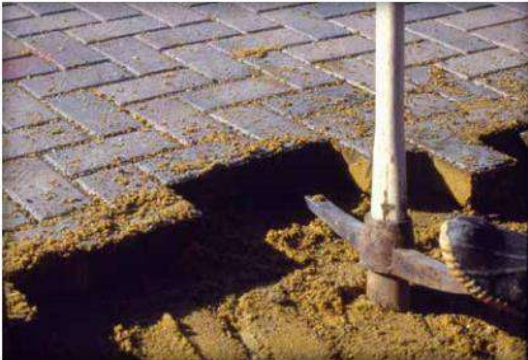
Figure 6. Prying out the remaining pavers
