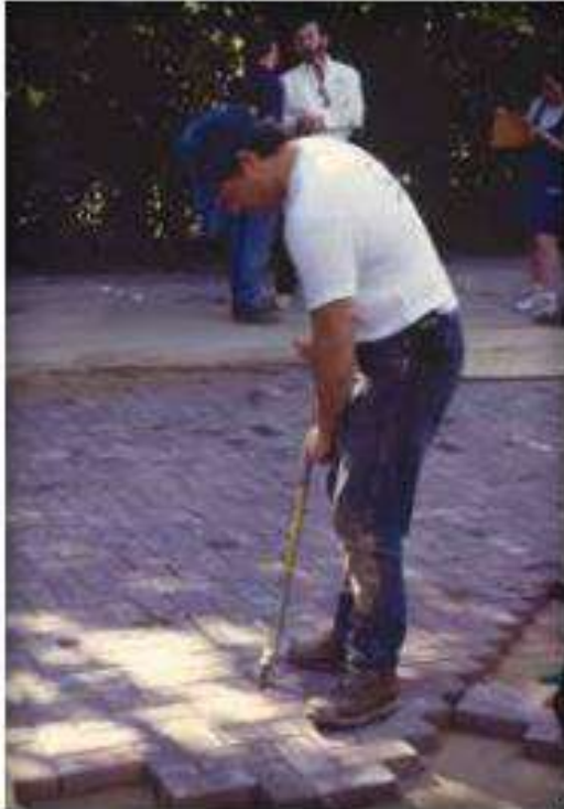
Figure 13. Adjusting joint spacing and alignment.
