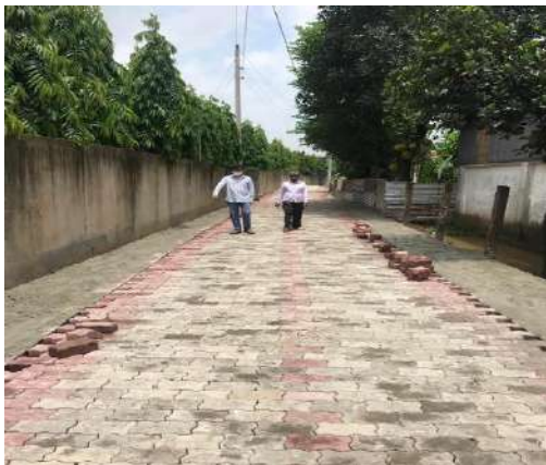
Figure: Ongoing Block Laying
