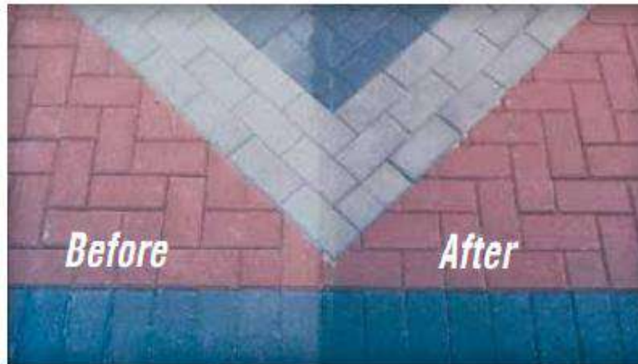
Figure 8. Before and after application of an acrylic sealer shows how it deepens the appearance of concrete pavers.
