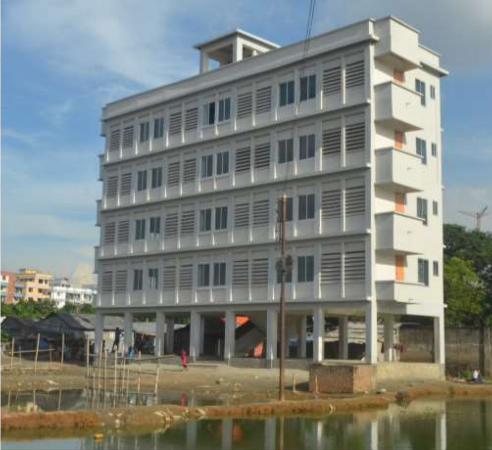
Multi-storied rural houses constructed using HBRI-invented construction technology
