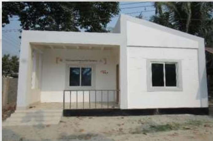
Resilient house for coastal areas using ferrocement channel and hollow blocks
