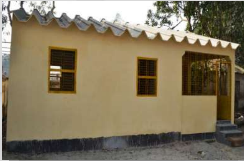
River Bank Erosion areas (Gaibandah)
