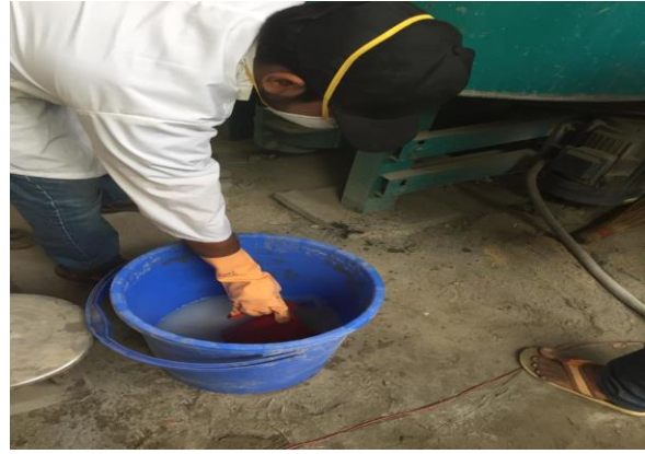
Fig-6: Mixing of Admixture with water
