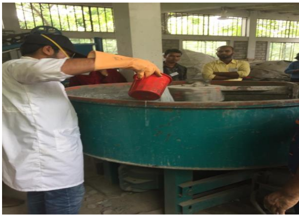
Fig-7: Admixture adding with raw materials
